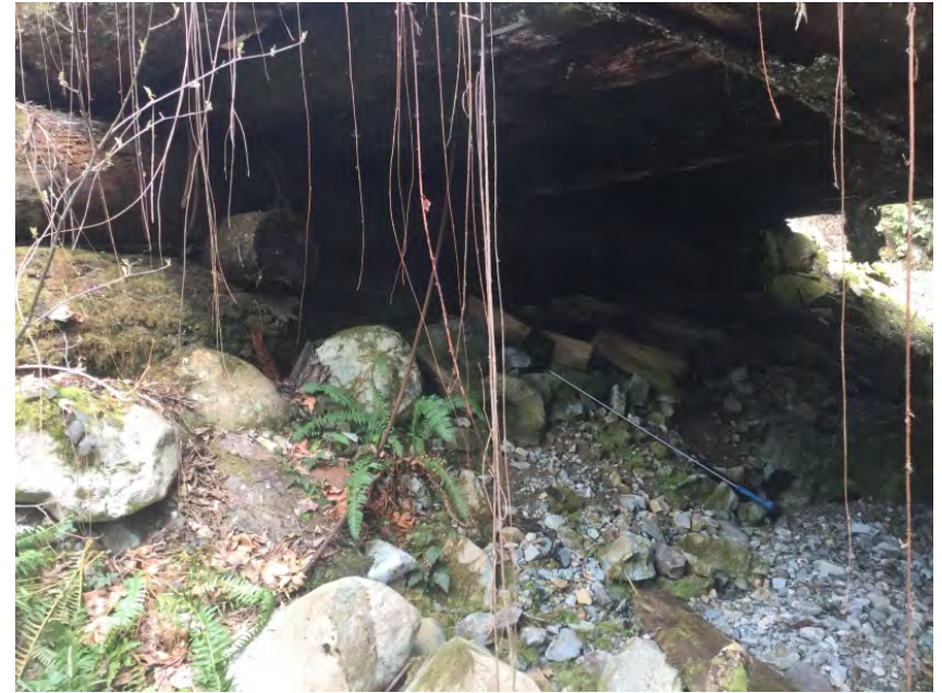
Right Bank Abutment when facing downstream
