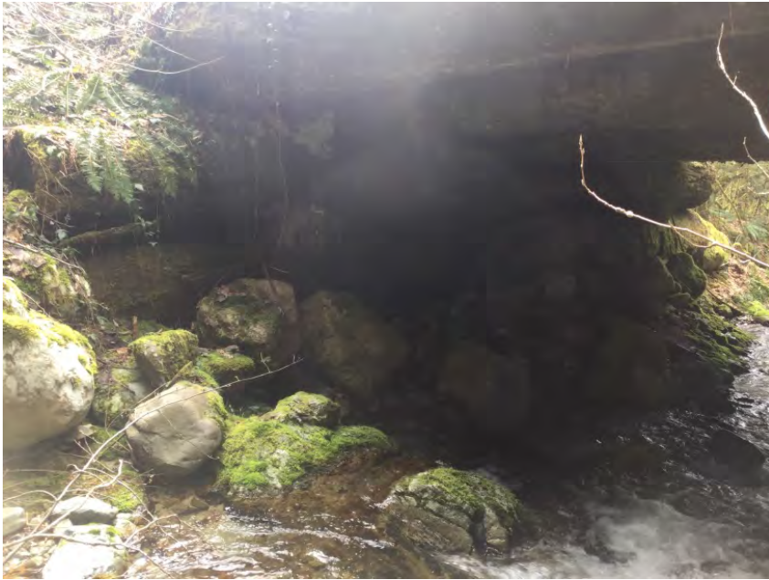
Left Bank Abutment when facing downstream
